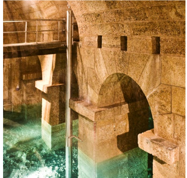
Kaiserbrunn source chamber
