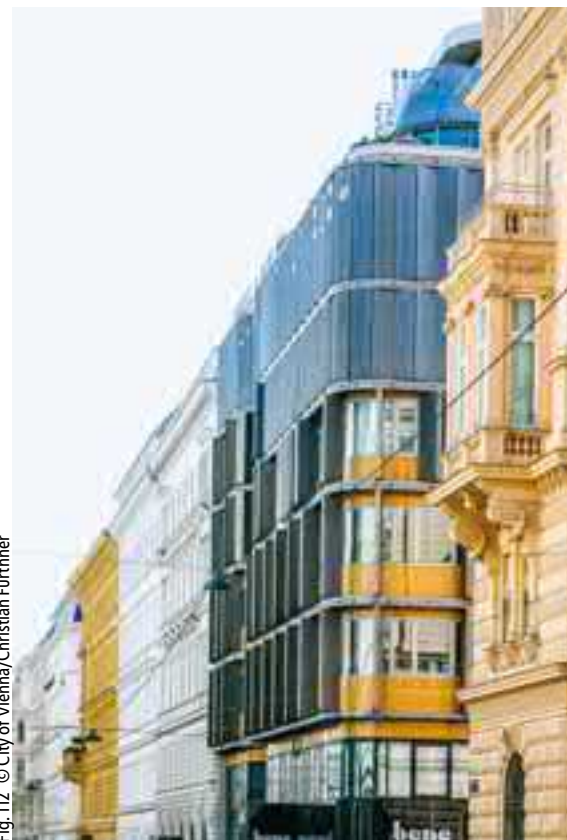
Bene office building in Neutorgasse (2010, Rataplan) (Fig. 112)
