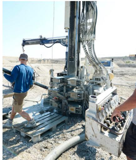
**Step 4:** On the right is the control console, which is used to operate the drilling rig manually. Up to two heat exchangers can be inserted into the ground in one day.
