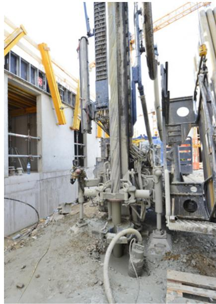
Renewable energy sources combined with concrete: A total of 30 borehole heat exchangers provide geothermal energy for efficient use in low-energy systems. © MA 20/A. Kromus
