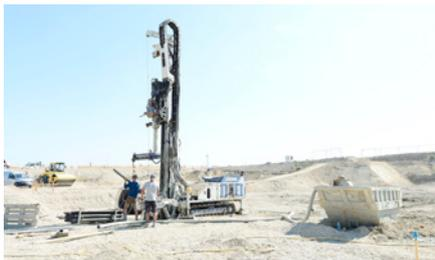
**Step 3:** The drilling rig installs the heat exchangers bit by bit. Over 9,000 lever movements are needed to lower one heat exchanger to a depth of 150 m.
