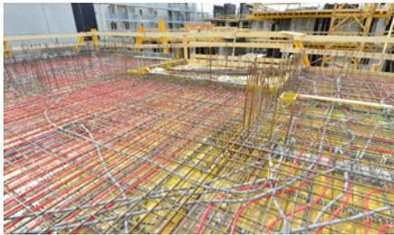
Hot or cold water is pumped through these pipes to heat or cool the building. © MA 20/A. Kromus
